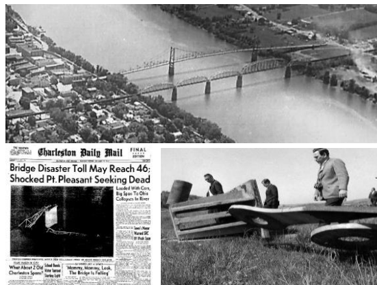
Figure 3.1: The silver bridge collapse at Point Pleasant and the structural part responsible for the failure.
