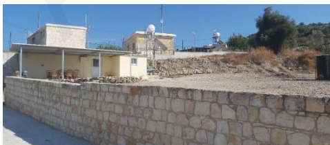
Figure 15. The Pelathousa slag heap in 2021 covered by a nice rock-façade.
