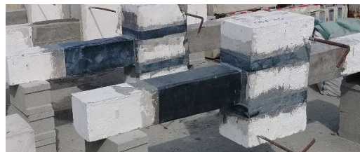
Figure 6. 7: Additional retrofitting of central stub and supporting part of the specimen
