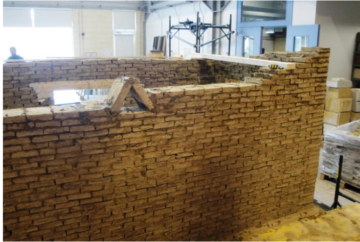
A3.6: Formation of triangular notch. A triangular notch 0.22 m wide and 0.18 m high was formed on the rear wall to simulate the ventilation notches encountered in local vernacular buildings.
