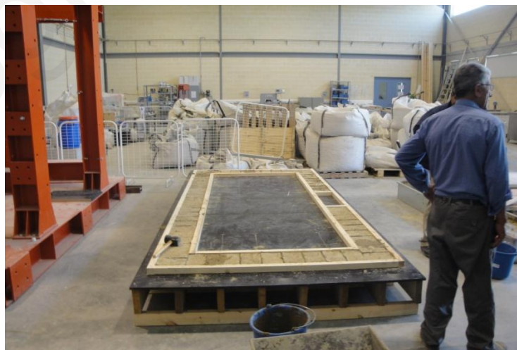
A3.2: Application of the first layer of adobes. Timber elements were installed at the perimeter of the first masonry course to constrain lateral movement at the base of the structure.
