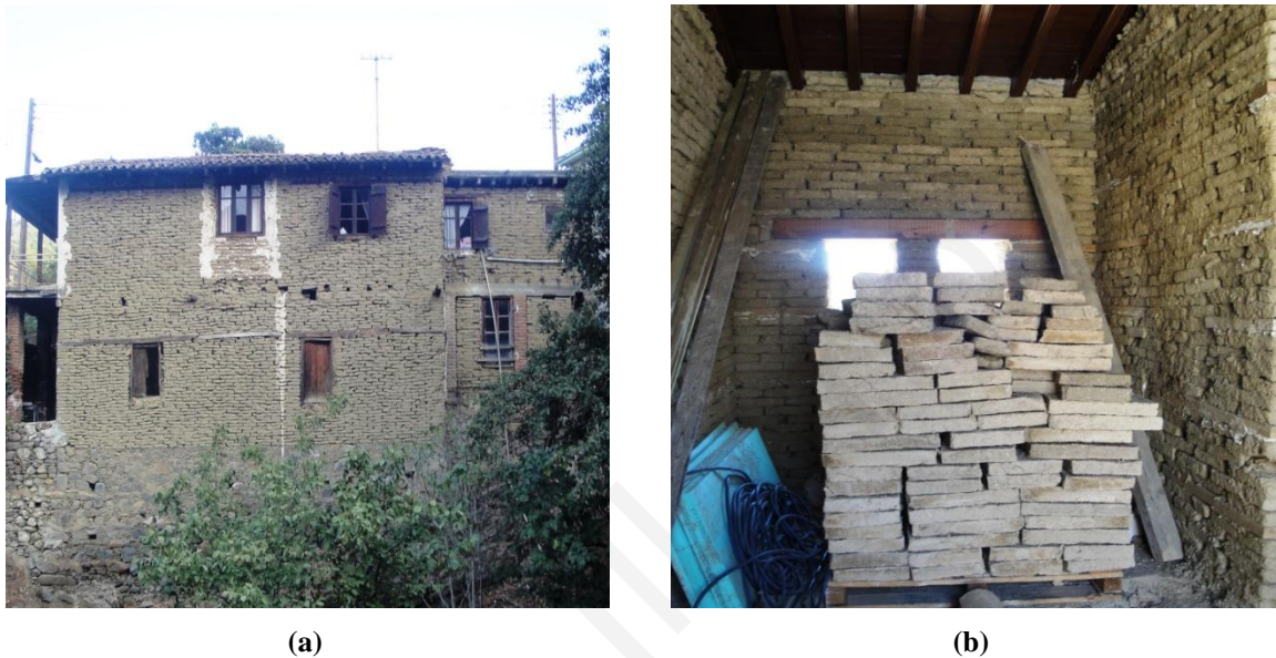
Figure 1.2: (a) Vernacular two-storey adobe masonry building in the village of Kakopetria, Cyprus. (b) Use of adobe bricks for the restoration of a traditional earthen dwelling in Cyprus.
