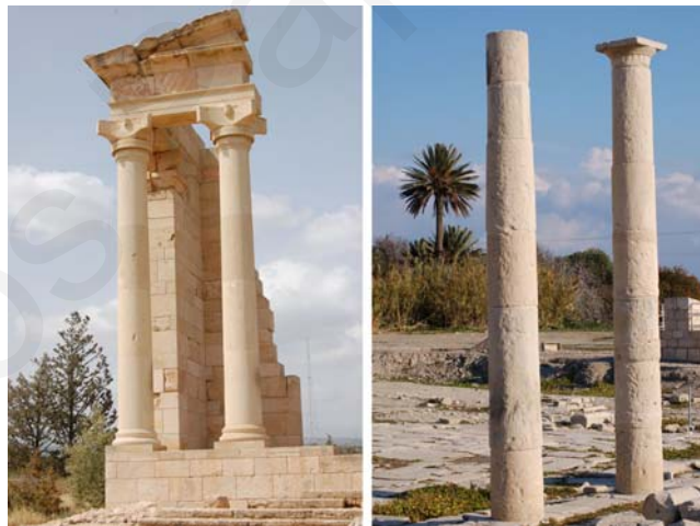
Figure 1.1. Ancient columns with an epistyle (Sanctuary of Apollo, Cyprus) and free standalone multi-drum columns (Amathus, Cyprus).
