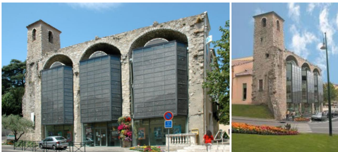
Figure 1. Integrated photovoltaics in the façade of historic building of Tourist Office in Alès (France) https://www.france-voyage.com/cities-towns/ales-9535/tourist-office-ales-5799.htm
