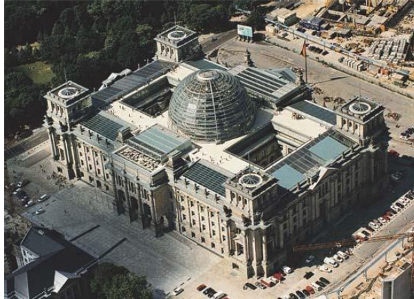
Figure 2. Photovoltaics elements on the roof of the historic Reichstag parliamentary building in Berlin https://www.webpages.uidaho.edu/arch464/Hall%20of%20Fame/Arch464/Spring2014/CS3/Reichstag%20Germany%201.pdf
