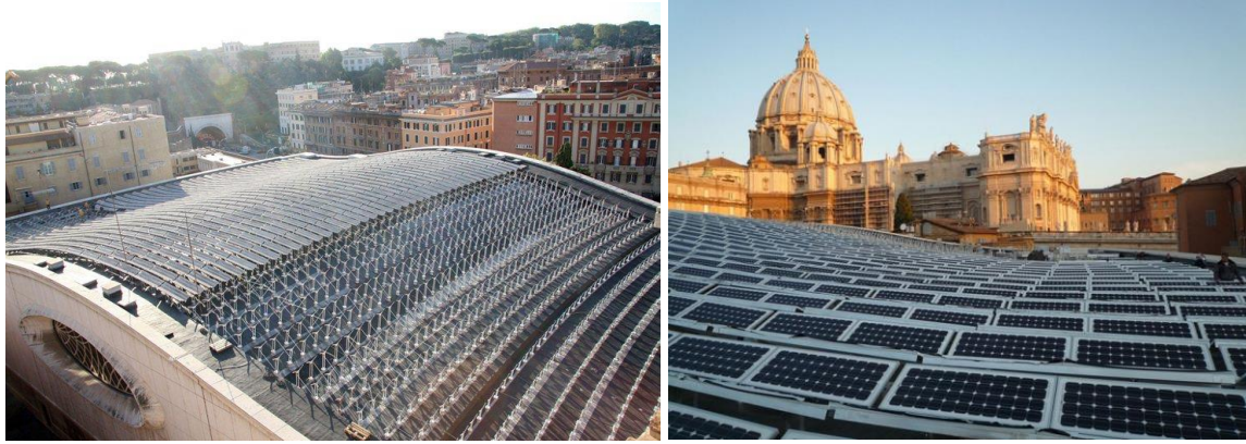
Figure 3. Photovoltaics panel on the roof of the historic Paul VI Audience Hall in Italy https://www.archilovers.com/projects/14001/copertura-solare-dell-aula-paolo-vi-in-vaticano.html#images
