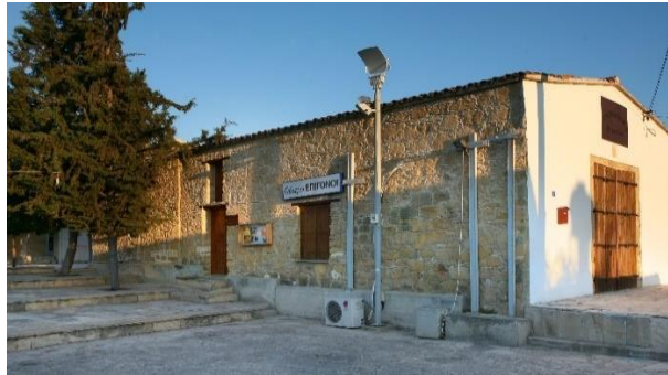
Figure 1. External view of the building under investigation, located at the traditional core of Aglantzia.
