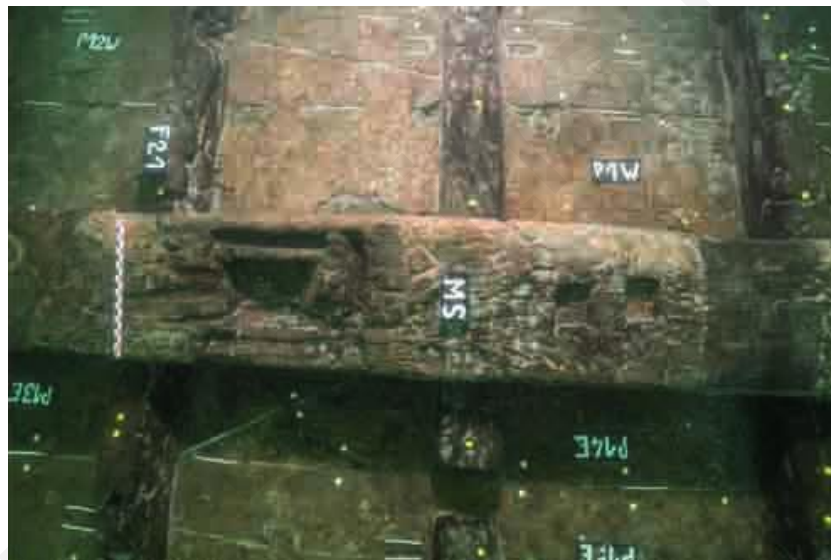
Figure 29: Caska 2: The main and the adjacent cavities for the mast, and the mortises for stanchions on the keelson/ mast-step (Rossi & Boetto 2020: 24, fig. 28c).
