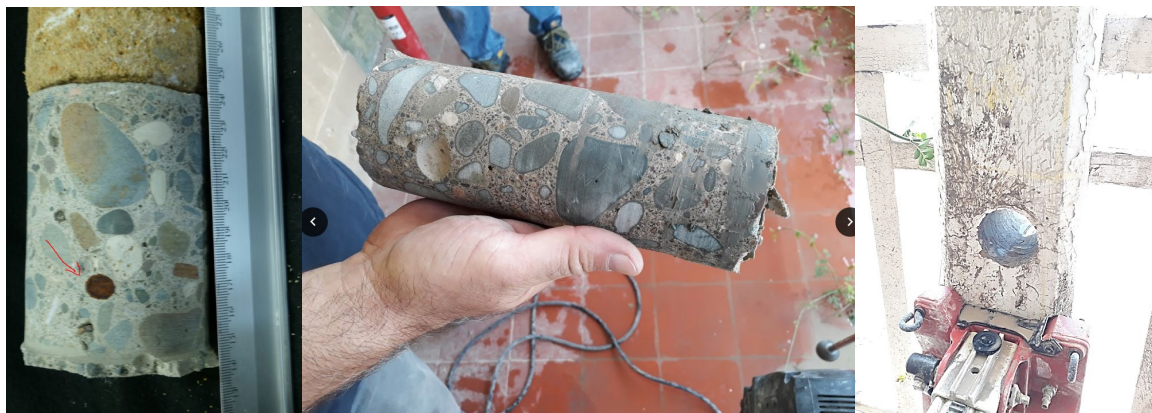
Figure 2: Left: Core sample taken from basement ceiling slab with reinforcement embedded in it. Middle: Core sample taken from column. Right: Location of core sampling from column.
