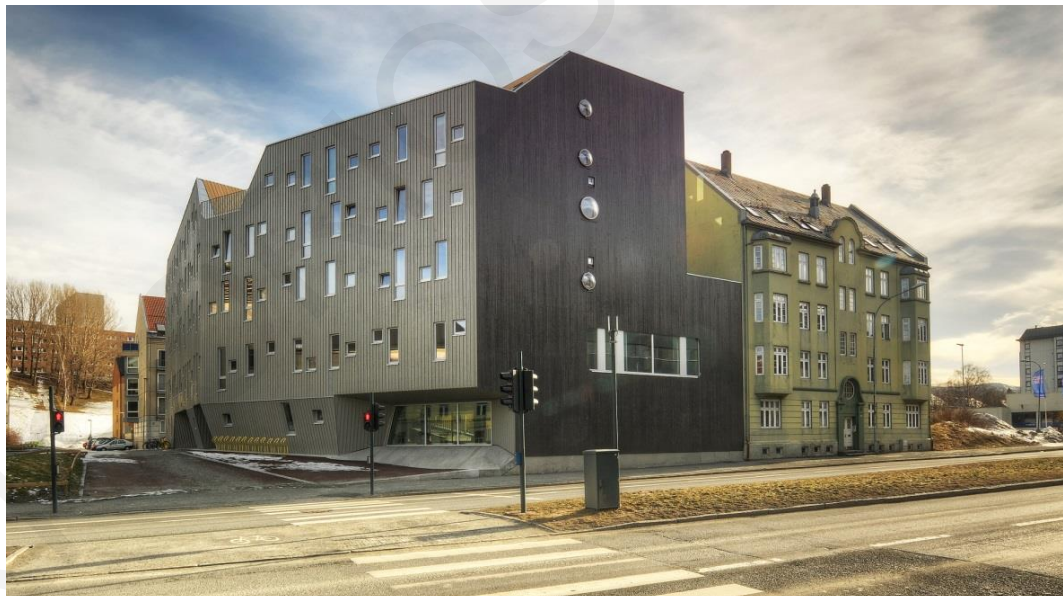
Figure 190: The winning project 'MySpace', a student's housing in Trondheim (Norway), is the outcome of a winning entry of European 9 by MEK Architects, Clara Murado, Juan Elvira and Enrique Krahe. The competition brief called for a student house between the Nidelva River and the main University Campus. The building has been nominated to the Statens Byggeskikkpris 2012, the Norwegian National Building Award and has won the Trondheim Kommune Energispareprisen (Energy Saving Prize 2012) (Murado & Elvira)
