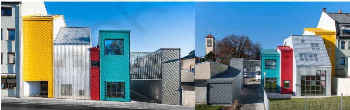
Figures 49, 50: The realization of the Haus der Tagesmütter (Gutiérrez-de-laFuente Arquitectos, 2015a)
