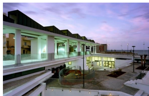
Figure 174: The first step of realization for the project 'Scenario for the Space Between': public square and rehabilitation center (European Europe)
