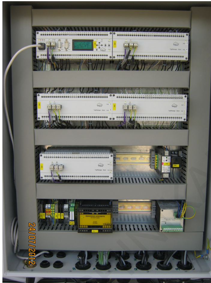
Figure 3.3: Delphin TopMessage data logger at the outdoor test site.
