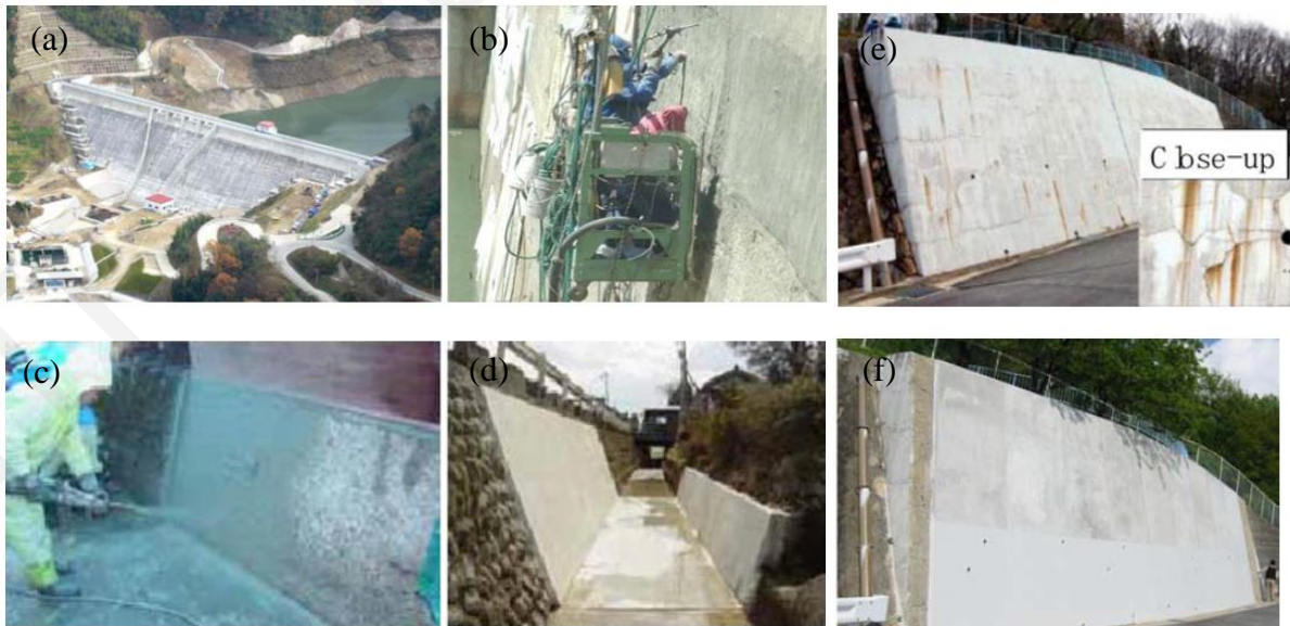
Figure 2.9 (a) Dam retrofitting application overview, (b) Direct spray construction, (c) and (d) Waterway structure, (e) and (f) Retaining wall retrofitting application [54]
