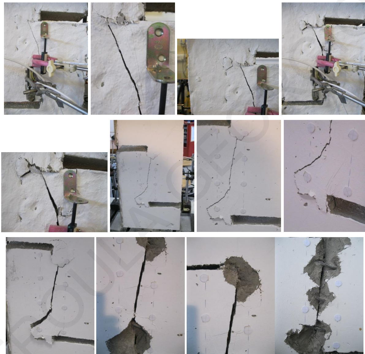
Figure 8.5: Crack sequence on both sides of a specimen without fiber but with steel reinforcement crossing the shear plane (Specimen F7-S1 or SHFRCC-S)
