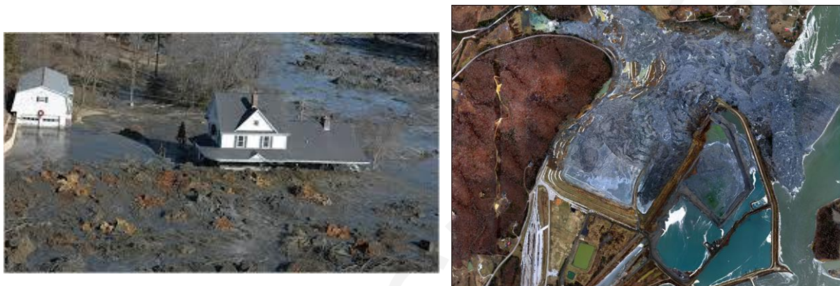
Figure 2.7: Dec. 22, 2008 a containment dike ruptured at Kingston Fossil Plant near Kingston, Tenn [33]
