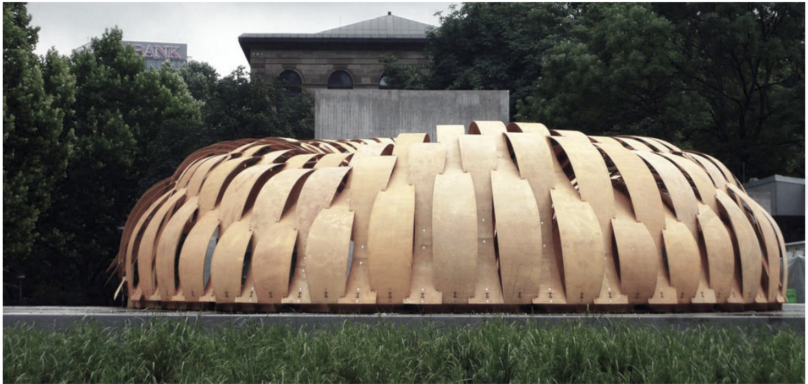
Figure 2.6 ICD/ITKE Research Pavilion, Stuttgart, Germany, 2010 (Lienhard, 2014)
