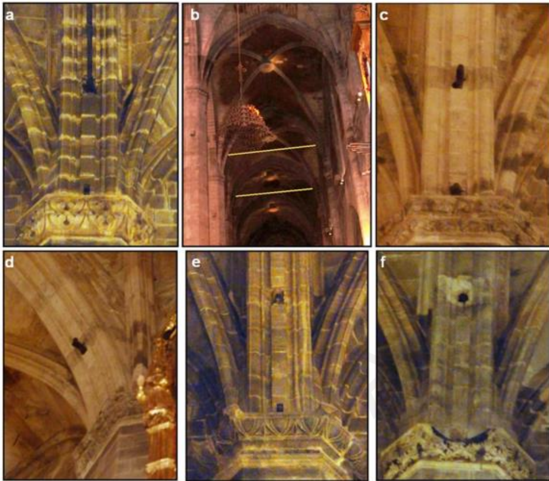
Figure 6 Dark spots and remaining hoops of the removed, temporary tie rods (Luca Pel à J. B., 2016)
