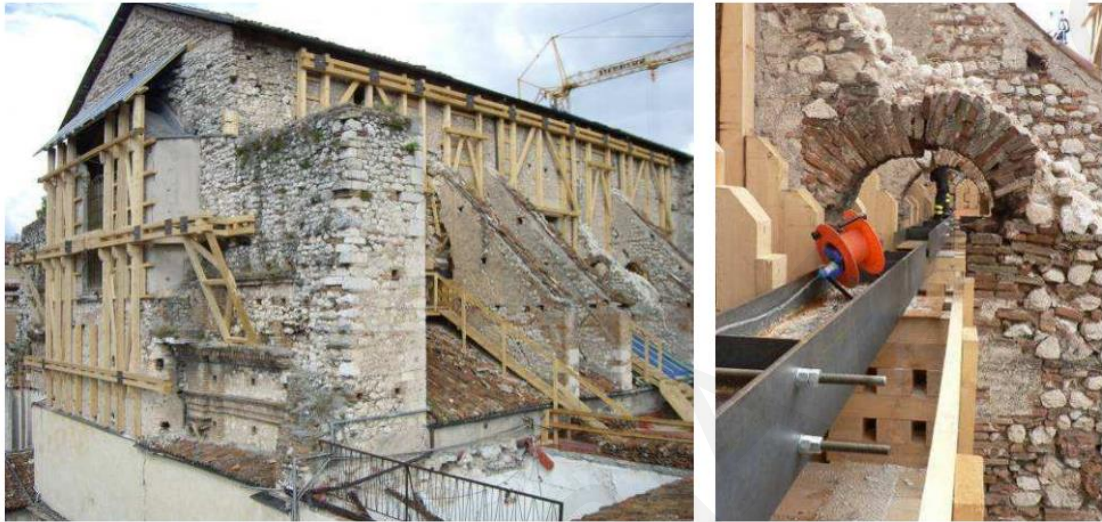
Figure 11 Santa Margherita restoration with metallic ropes
