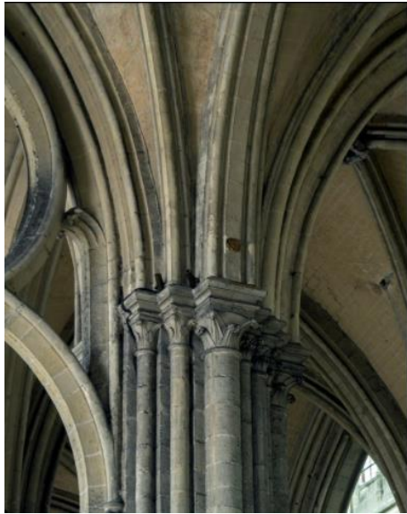
Figure 7 Signs of Wooden tie rods in Amiens Cathedral (Media Center of Art History, 2020)
