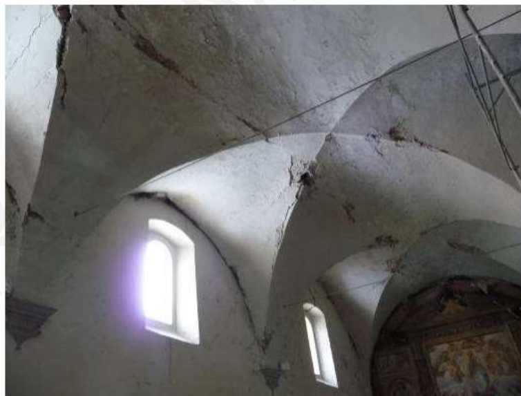
Figure 12 Beata Antonia tie-rods placed after intervention
