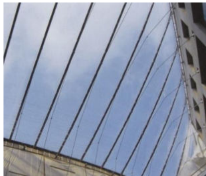
Figure 3.13 ETFE roof from below and inflated cushions fixed to a cable structure that easily deform to define the desired warped surface in an industry building
