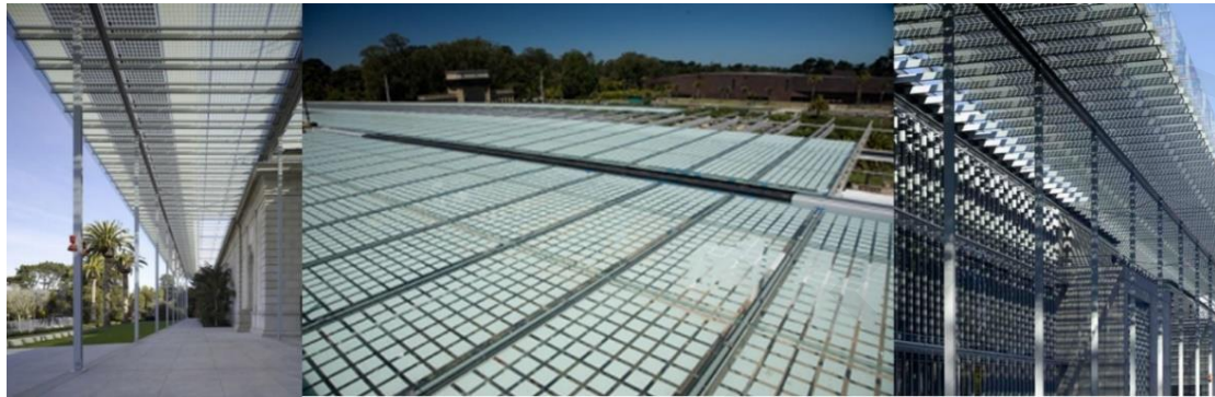
Figure 15. Semi-Transparent PV Canopy Side View, Top View, View from Below (starting from left to right) [13], [14].
