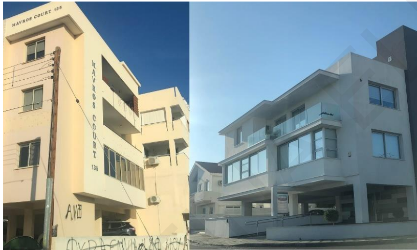
Figure 1. Examples of Closing up the Veranda Space on Existing Apartment blocks in Cyprus.
