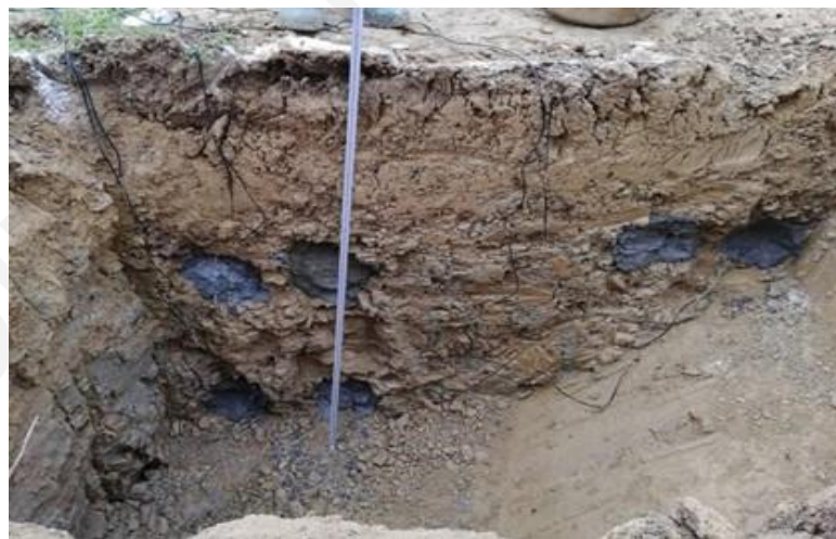
Figure 34. Installation of ground sensors in Site 3
