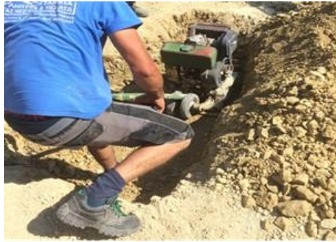
Figure 18. Backfilling and compacting test pit 1.
