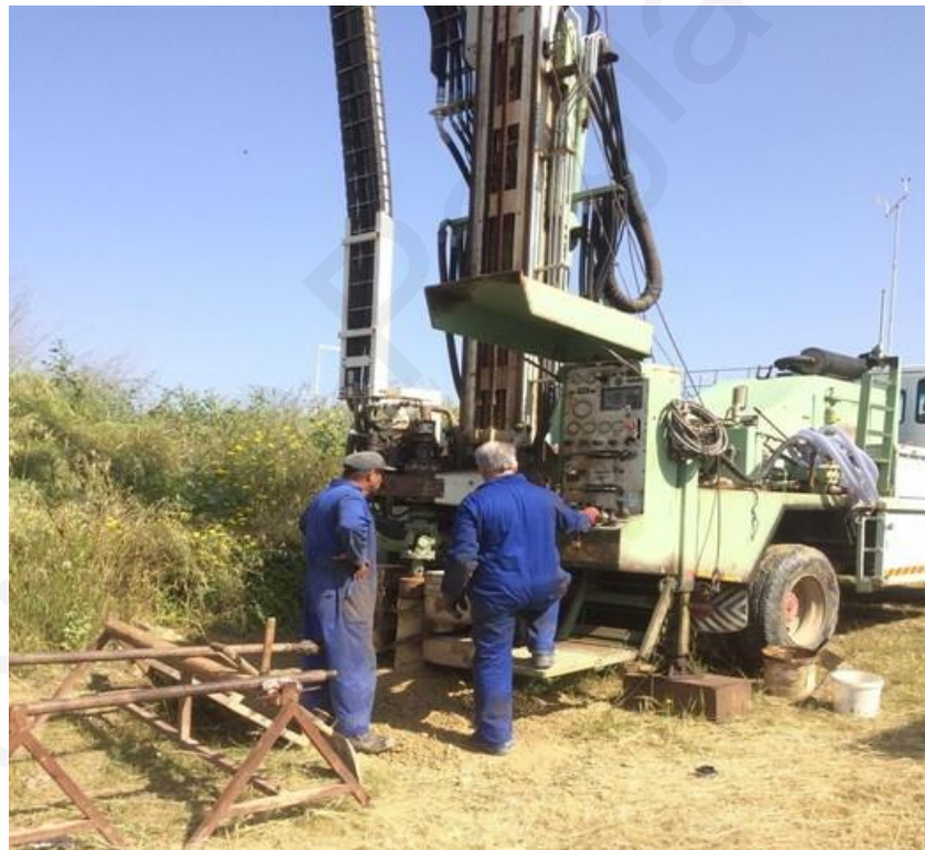
Figure 21. Exploratory drilling at Site 2 (BH2).
