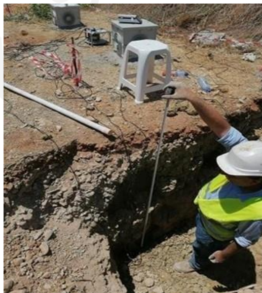
Figure 25. Field work for the installation of sensors at Site 2.
