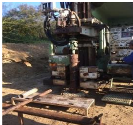
Figure 11. Drilling at Site 1 (BH 1)
