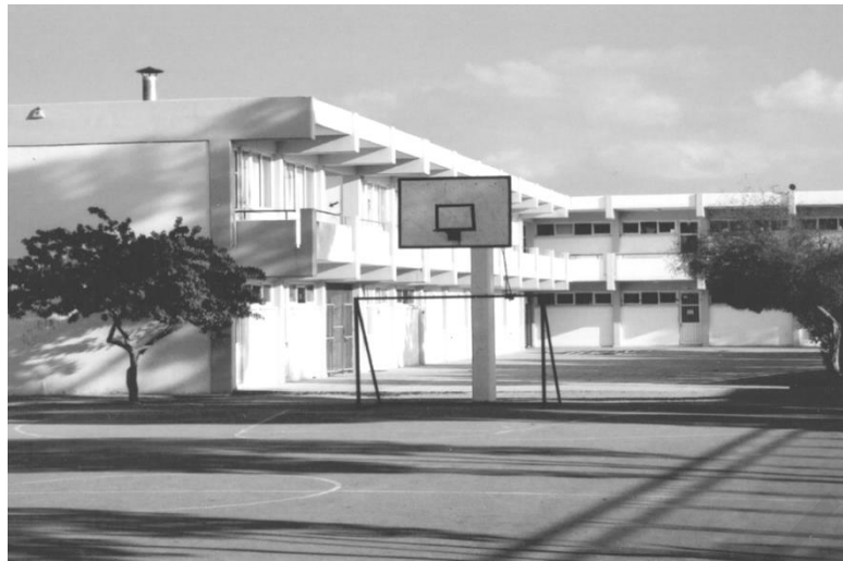
Figure 10.3. Secondary School of Stavrou Strovolou (Nicosia 1992), Technical Services of the Ministry of Education, Culture, Sport and Youth.
