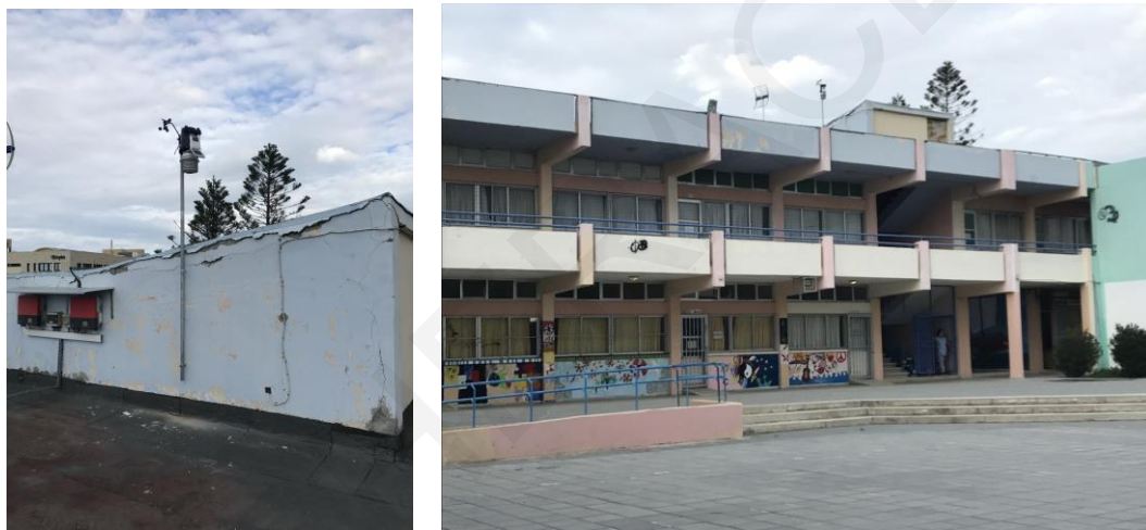
Figure 11.6. Outdoor weather station installed on the building's roof, at a height of 10m above street level, i.e. 4 metres above the regular height of buildings.
