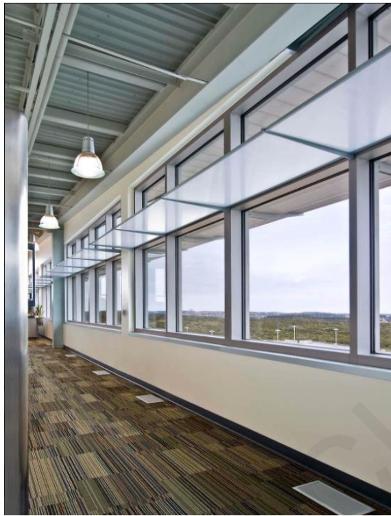
Figure 7.9. Reflectors and lighting shelves [400].
