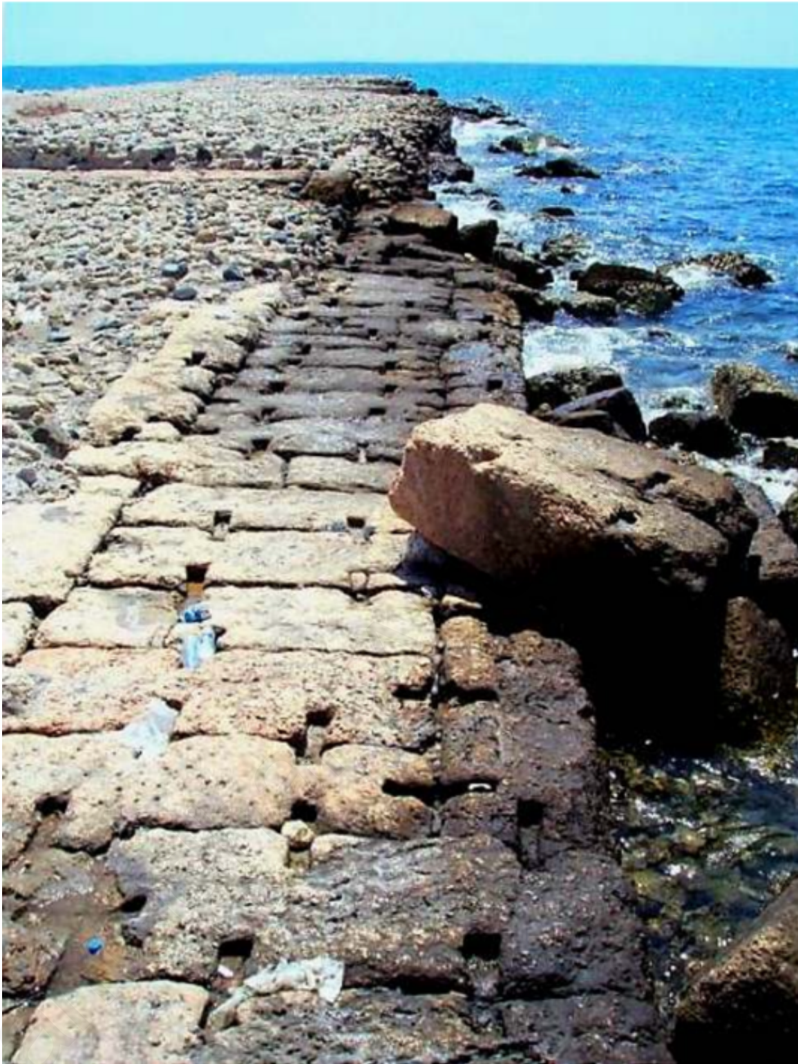
Figure. 32. The ashlar wall that containing marine concrete at Soli-Pompeiopolis breakwater/mole. The surface stones were fastened to each other (Oleson, 2014, 517).
