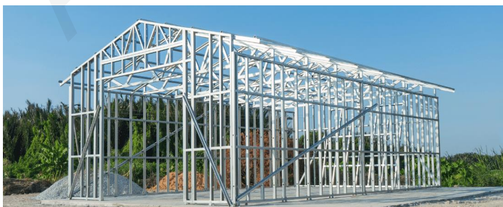
Figure 1.1: Cold-formed steel members in construction (CSSBI, 2021).
