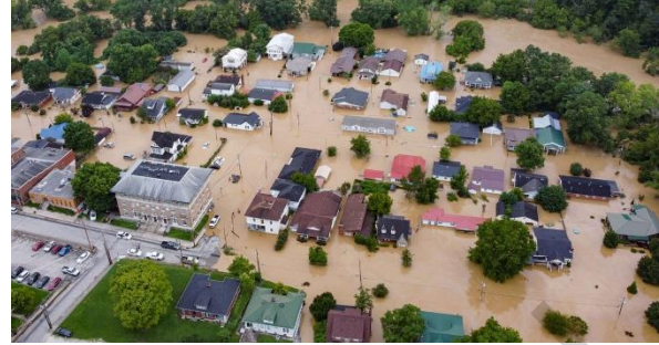
Figure 3: Flood-caused disaster Source: https://shorturl.at/aqsR3
